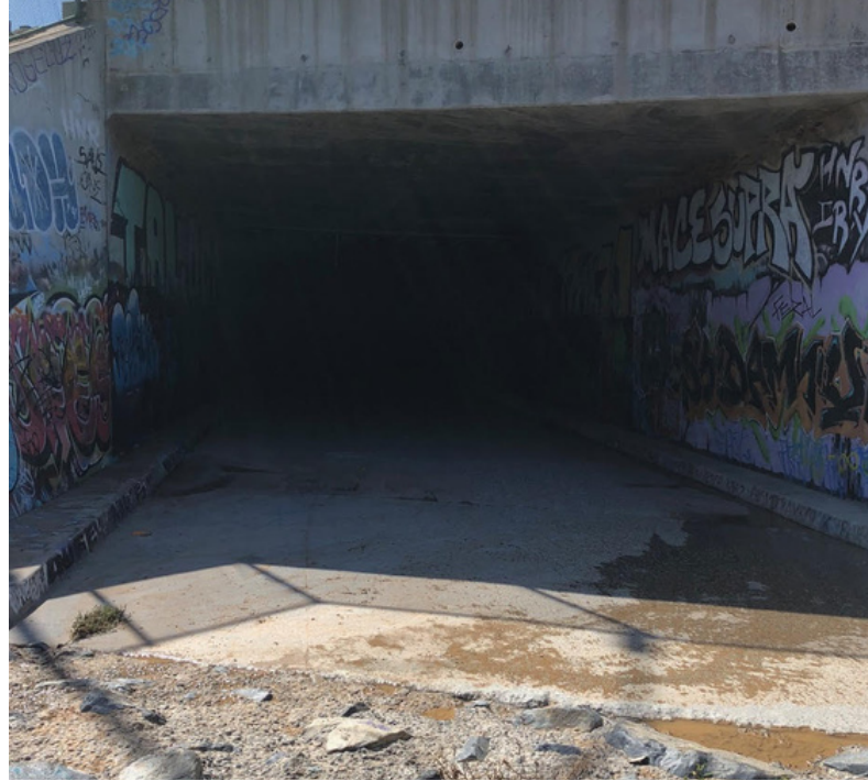
CULVERT AT THE I-5 PREVENTS ANIMAL MOVEMENT UNDER FREEWAY
