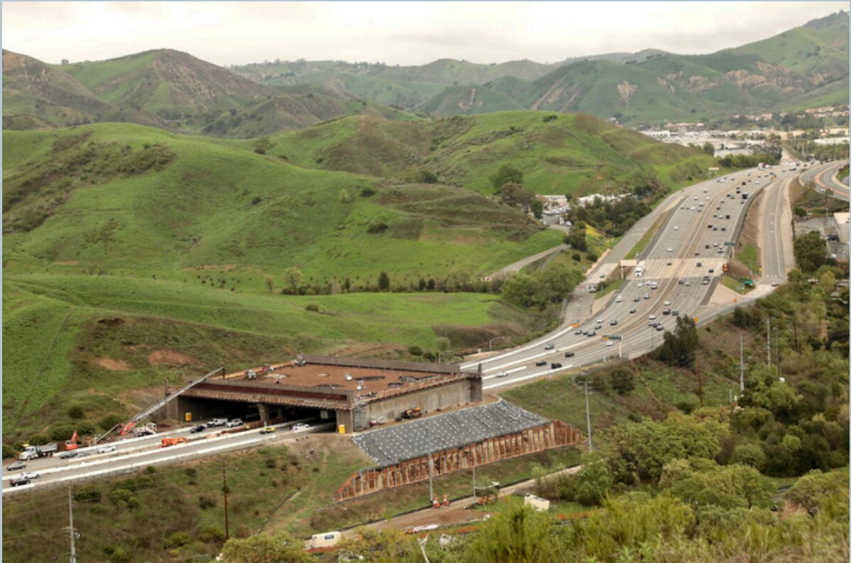
Photo of the Wallis Annenberg Wildlife Crossing in Ventura County in March 2025 when construction crews first began laying soil.
